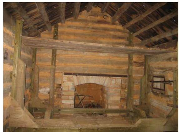
*Figure B-5* View of added bracing inside cabin
