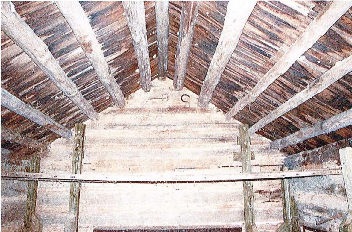
**Figure 5** The roof framing consists of log purlins set parallel to the ridge.
