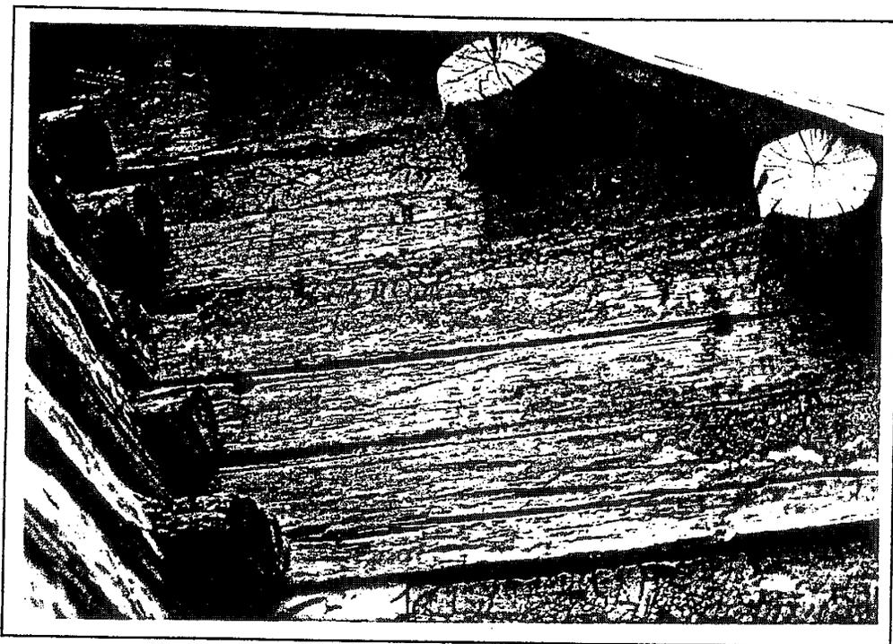
Figure 10. Auger holes located in the west gable.
