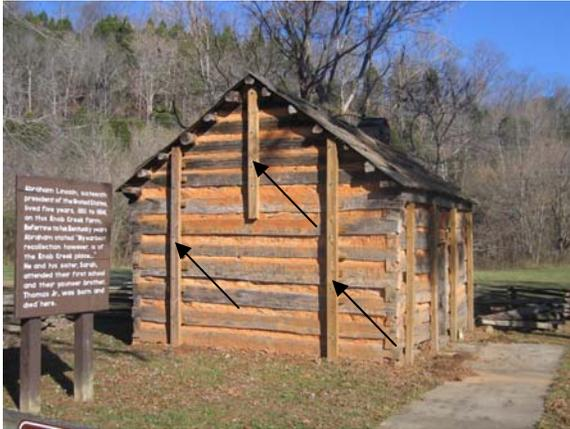
**Figure C-4** Cabin southeast oblique, added vertical bracing noted
