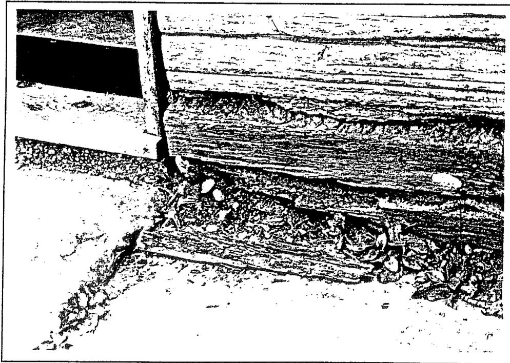
Figure 7. Detail of deterioration of sill at doorway.
