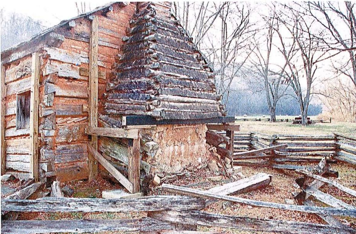
**Figure 4** The fireplace enclosure has partially collapsed.
