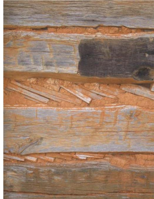
**Figure C-5** Detail of logs and chinking
