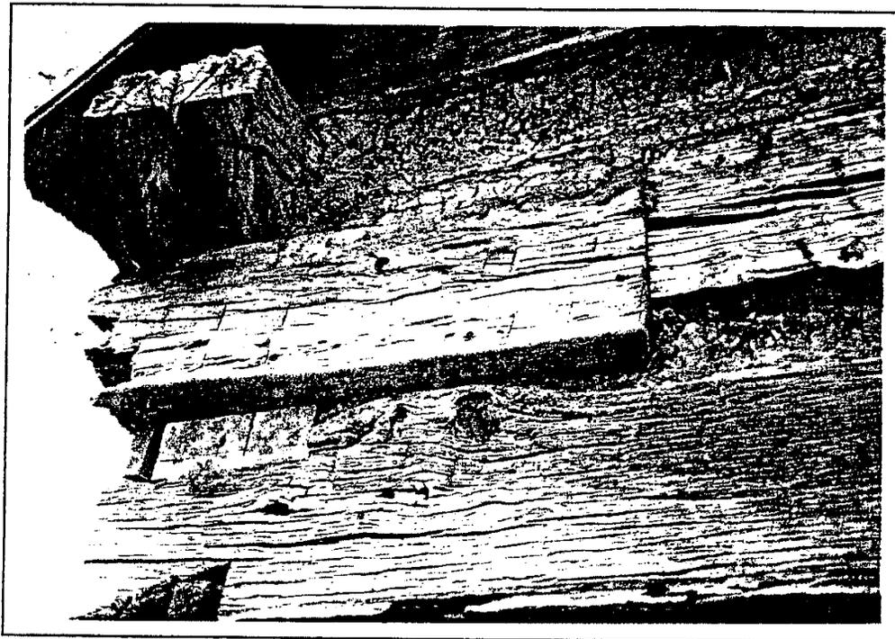
Figure 15. Closeup of spliced section of eave beam.
