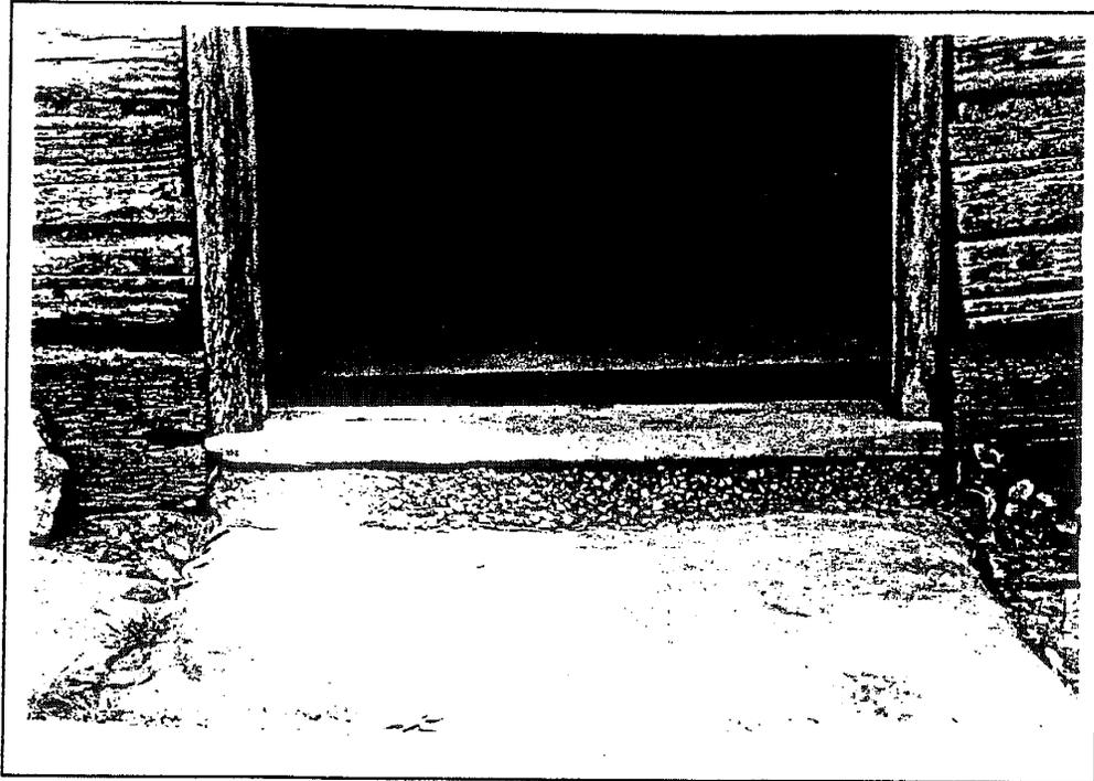
Figure 6. View showing cut in sill.
