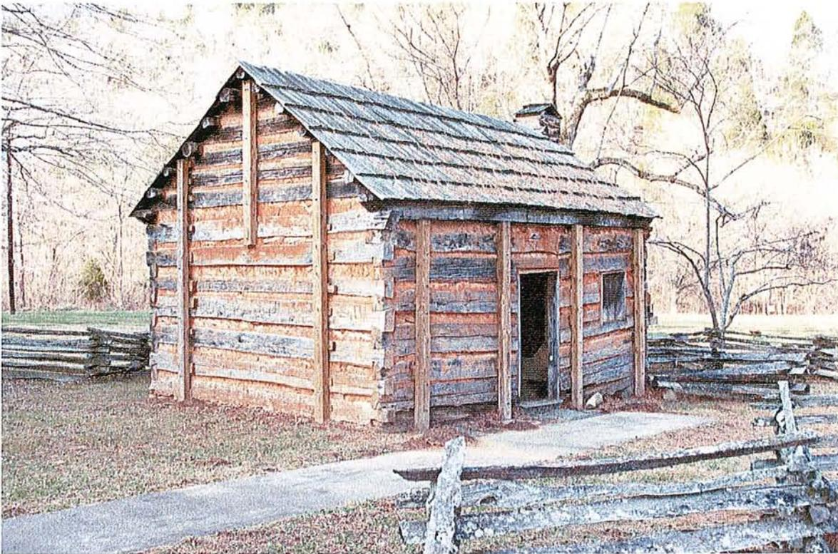
**Figure 1** The Boyhood Home has been braced to prevent collapse.
