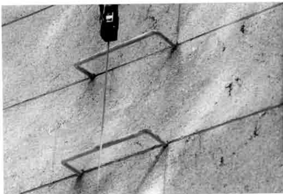
Steel rungs appear to be rusting. Extent of deterioration has not been determined. There is some outward movement in at least one rung.
