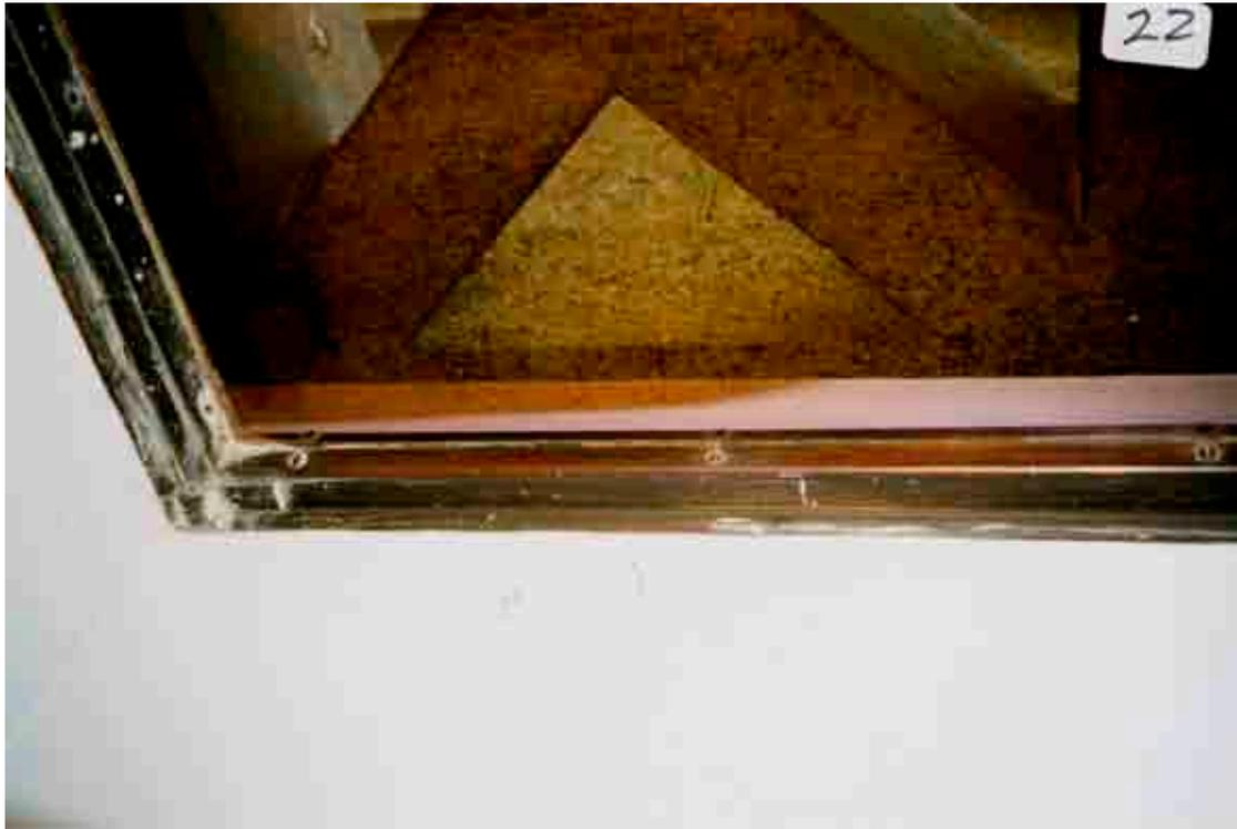
Figure 9. View of typical east/west wall window, showing bronze interior frame. Note sloppy paint work.
