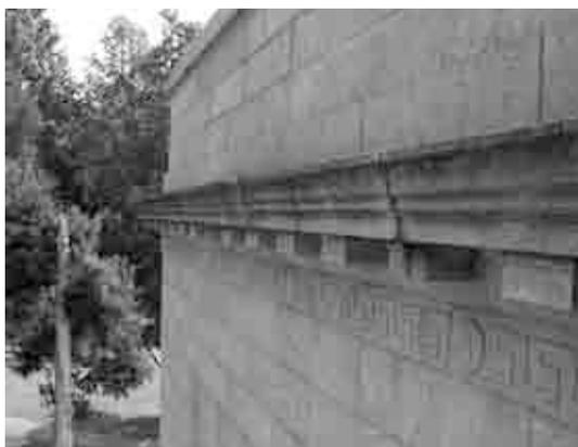
Granite wall parapet (Dirt and mildew buildup on cornice)
