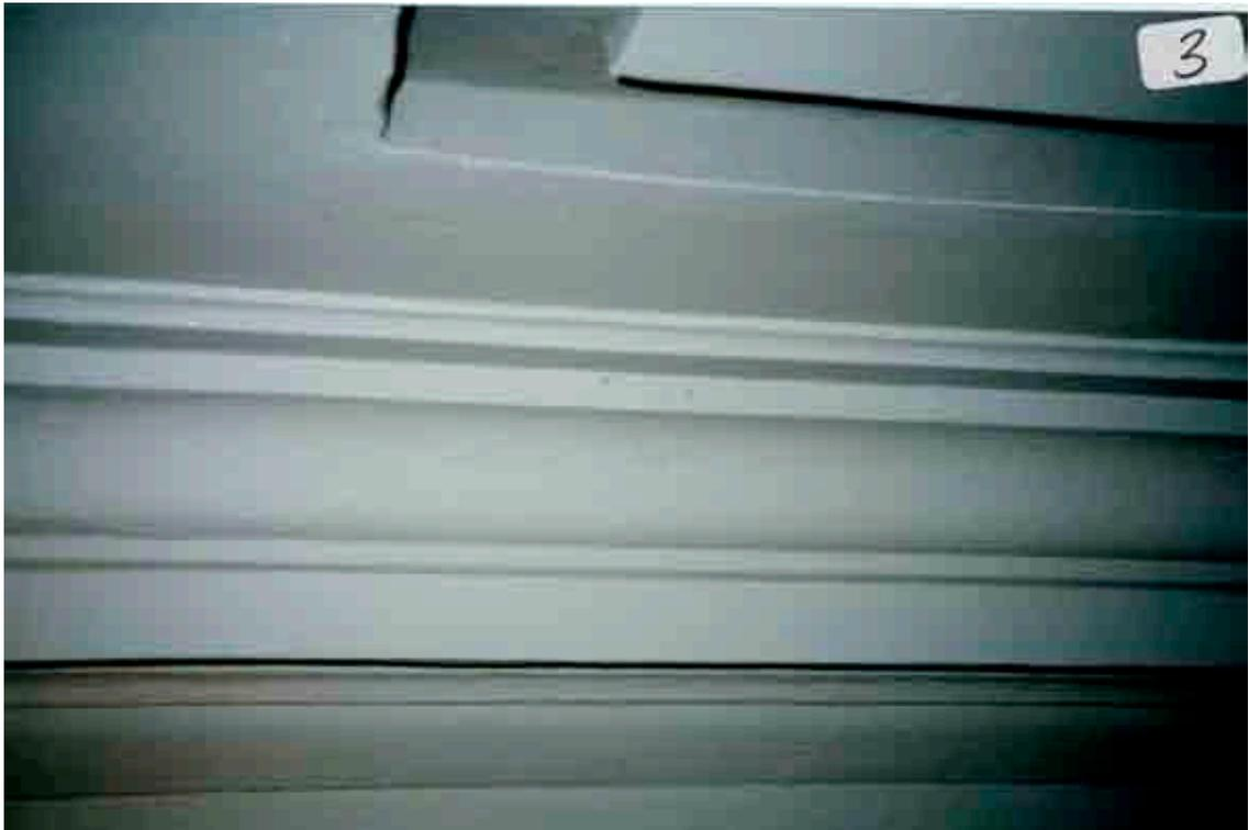
Figure 3. View of crisp profile of cornice which has not been repaired, or, if repaired, was done using a proper template.
