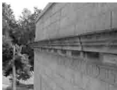
*Dirt and mildew buildup on cornice at north elevation (above and below)*
