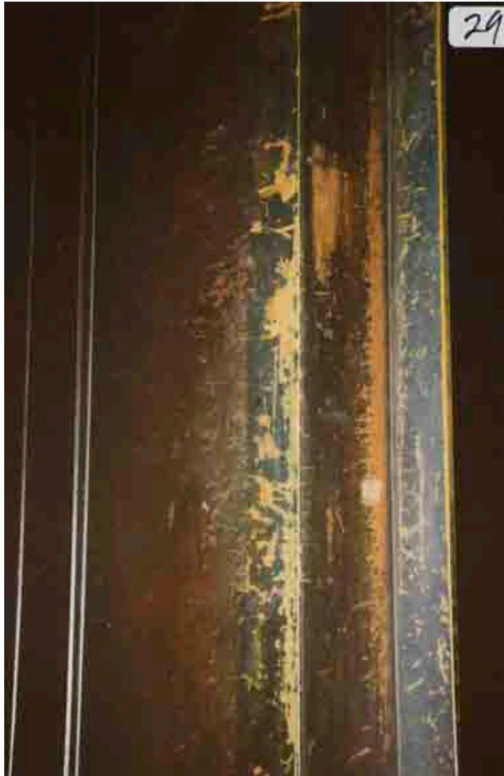
Figure 10. Severe deterioration of coatings and patina, typical on edges of all bronze doors.
