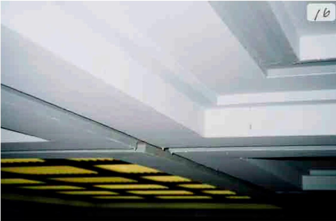
Figure 6. View across ceiling showing drips (“stalactites”) of sprayed-on recent thick coating.
