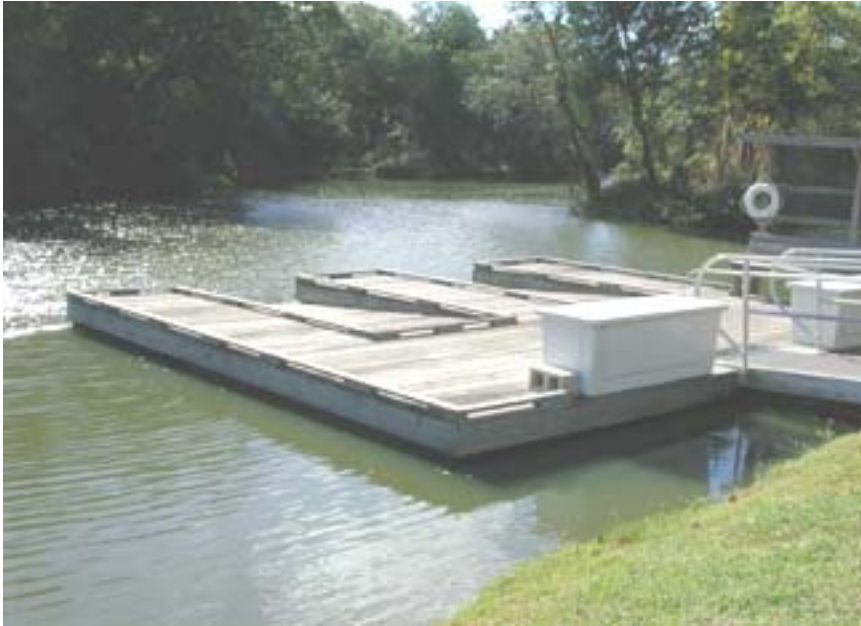
Photos 3C, 3D: ADA accessible wooden floating launch has two tapered ramps that allow canoes to slide up onto the deck
