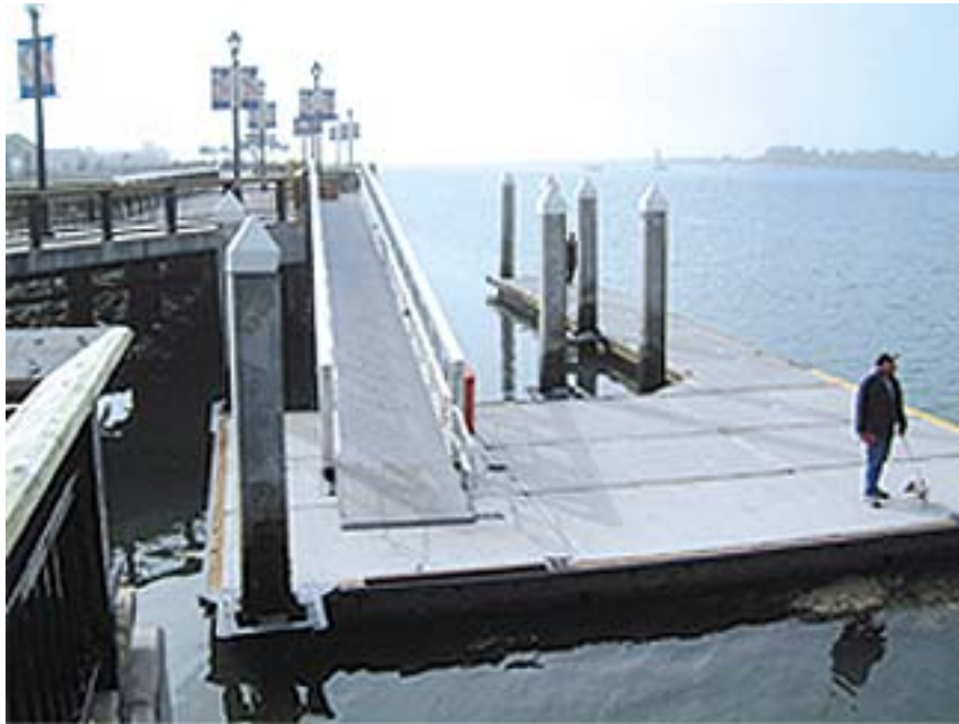
Photo 3E: Aluminum gangway serves as a ramp to floating launch
