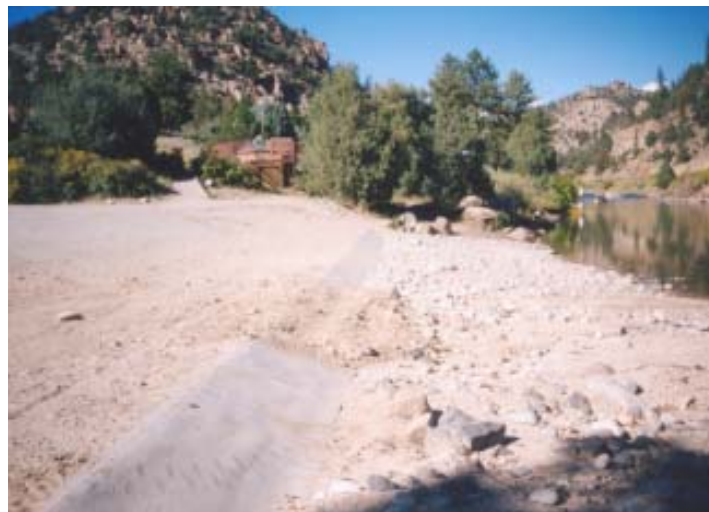
Photo 8M: Concrete strip helps to divert flows away from launch site
