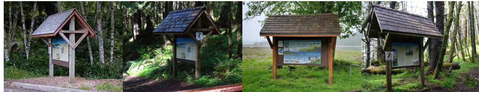
Dimensional Wood | Gable Roof | Shingles
