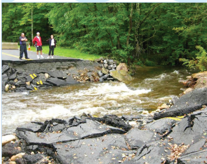
The Town of Becket used the opinion of probable costs and conceptual designs, funded by the Committee, to leverage an additional $399,000 in grant funds to replace this road-stream crossing with a fish-friendly, flood resilient structure. The road-stream crossing had washed out two times in less than six years.
