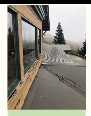
Window damage from water intrusion
