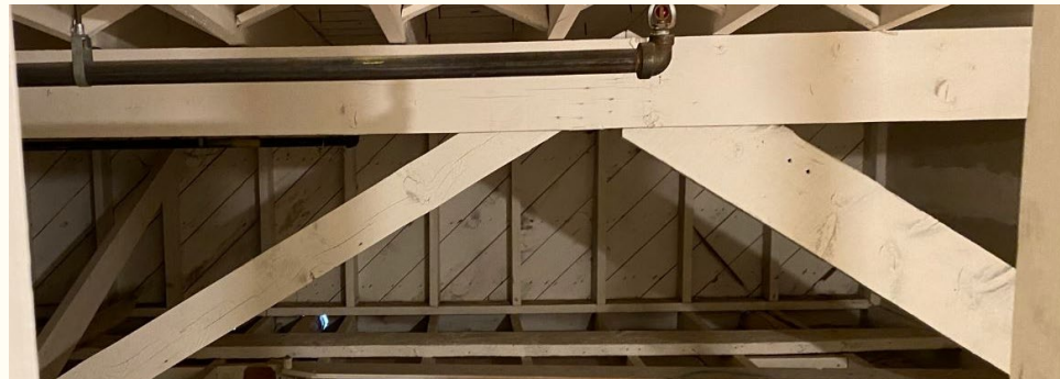
View in the attic, Poor Building envelope improper seismic diaphragm & connectors
