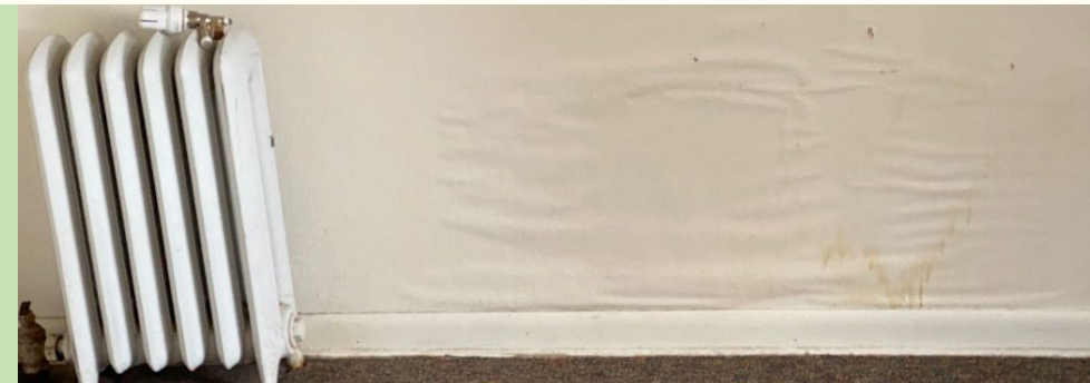
Typical water damage due to high humidity, a result of being built on top of active geothermal ground
