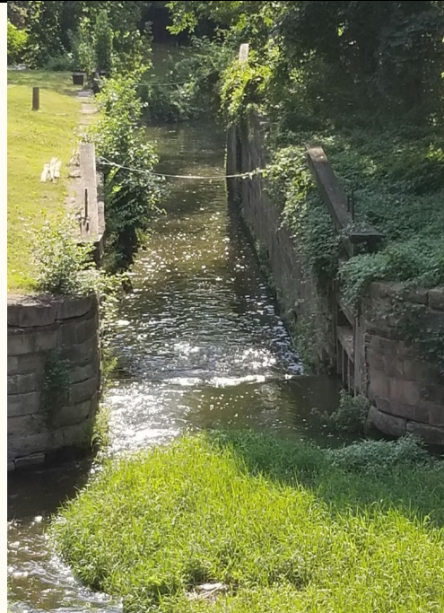
Lock Walls Repair Walls, Repoint Joints, Pressure Grout Stone Mass
