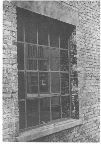
or deteriorated metal pieces. At the same time, racked metal sections, especially the center-pivoting hopper units, were realigned by applying heat and pressure. All the metal was then painted with an anti-corrosive paint.
