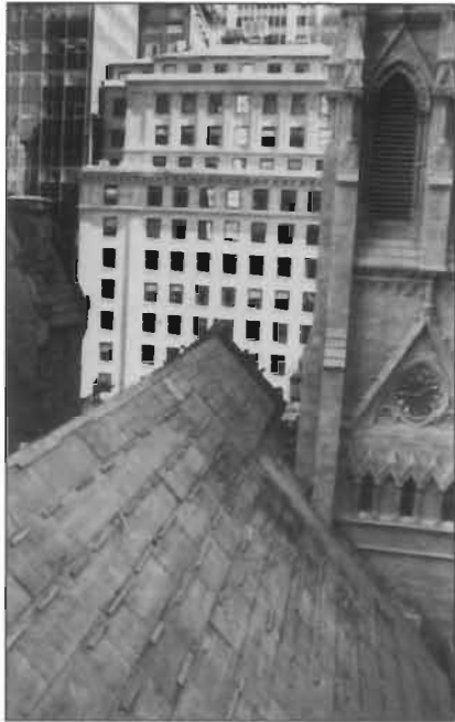
▲► The roof and stained glass windows of this historic church have been appropriately covered with plywood as a protective measure during construction of a new building on an adjacent lot.
