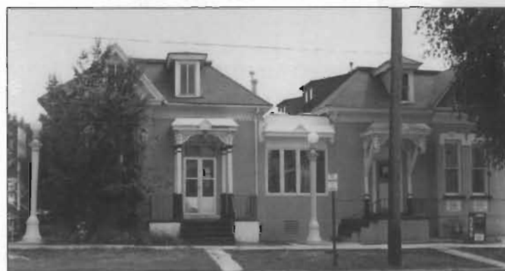
Two small Victorian cottages, above, were connected to provide additional floor space in a commercial rehabilitation. The inappropriate infill connector, below, is on the same plane as the historic facades, essentially making the two cottages appear as one building. If the new infill had been substantially set back from the facade, the distinct form of each cottage would have been retained.
