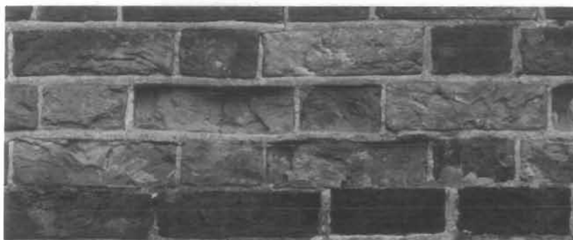
Too hard and inflexible a mortar has caused this soft, 18th century brick to spall.
