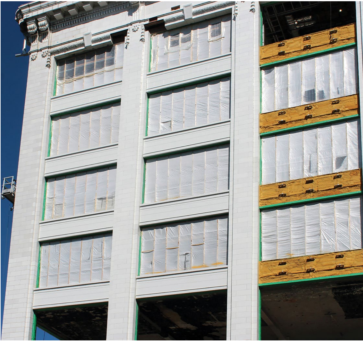
Figure 18. Missing historic terra cotta spandrel panels on all floor levels were recreated utilizing glass fiber reinforced concrete (GFRF) replacements. New spandrels were fabricated as individual components and attached with metal clips between historic terra cotta piers. Photo: Kris Frail, Dewberry.
