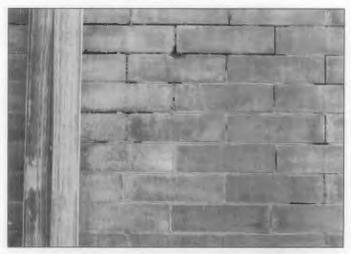
Figure 2. Much of the mortar on this building has been leached away by water from a leaking downspout. The downspout must be replaced and any other drainage problems repaired before repointing. Photo: Robert C. Mack, FAIA.
