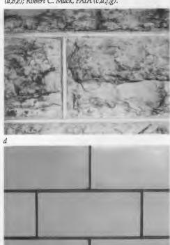
application of a raised joint or lime putty joint on top of flush mortar joints (Fig. 20). **Penciling** is a purely decorative, painted surface treatment over a mortar joint, often in a contrasting color.
