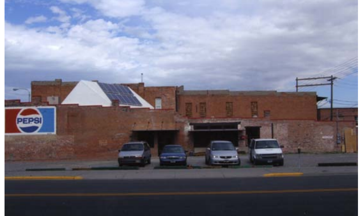
The addition of a large rooftop monitor featuring skylights on the front slope and solar panels on the rear slope is not compatible with the historic character of this small, one-story commercial building.
