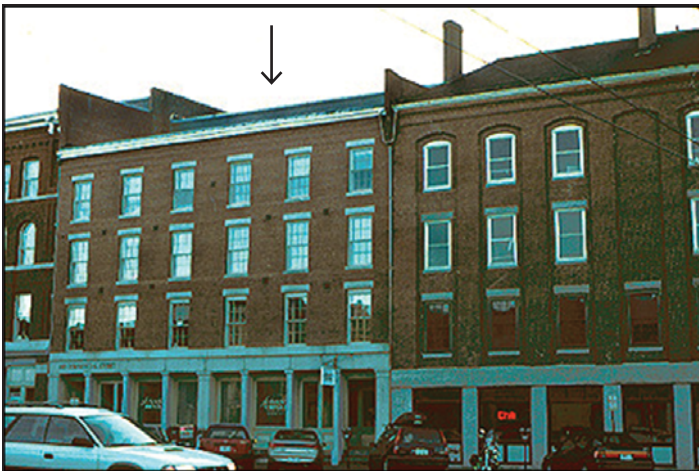
Mid-19th century commercial building with rooftop addition as it appeared after rehabilitation (center).
