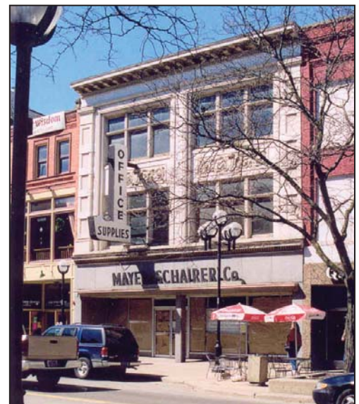
Three-story commercial building prior to rehabilitation.
