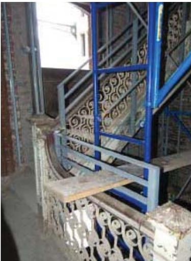
Accordingly, a more compatible (and more refined) supplemental railing was designed consisting of only two, much thinner rails supported by posts capped with finials. The revised design meets the Standards.
