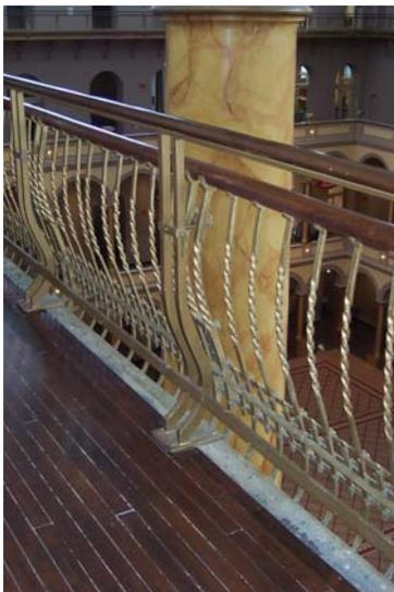
**Application 5** (*Compatible Treatment*): When this 1882 building was converted into a museum and offices, it was necessary to modify the height of an unusual wrought iron railing that encircled the atrium at the fourth floor level. To satisfy code requirements, an additional painted-metal railing was installed on the inner side that followed the contours of the historic railing. This appropriate design meets the Secretary's Standards.
