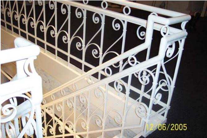
*Left: This sensitively executed modification provided the necessary height to this elaborate metal stair railing.*
