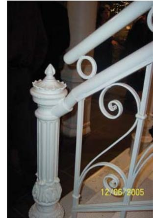
**Application 4** (*Incompatible treatment*): Prior to rehabilitation, this finely-detailed wood railing in a 1890s Victorian house was lower than allowed by code. As a result, it was modified by attaching a new pipe-metal railing next to the original railing. This highly visible change does not meet the Secretary's Standards because it diminishes the character of this important interior feature.
