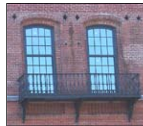
Left: Detail of the fire escape before rehabilitation. Right: Detail of the fire escape after its conversion to a balcony during rehabilitation.
