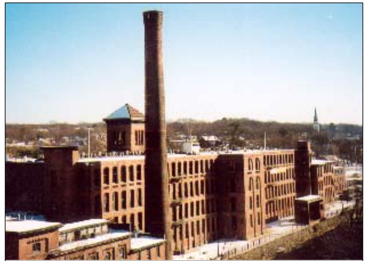
Many historic mill buildings that are being converted for residential use retain their historic fire escapes.
