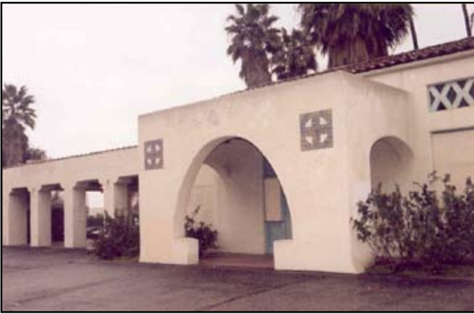
Exit leading to train platform before rehabilitation.
