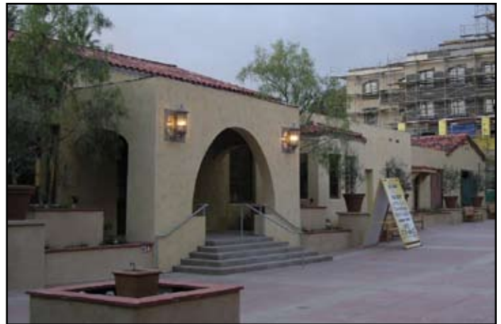
Exit with new steps to former train platform after rehabilitation.
