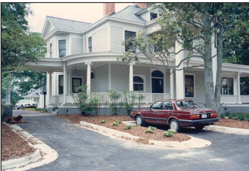
The new parking lot completes the drastic alteration of the setting. The second relocated structure (C2) can be seen through the porte-cochere at left.
