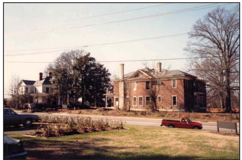
Turned 180 degrees, the moved building (B2) faces the historic one from a distance of 60 feet.
