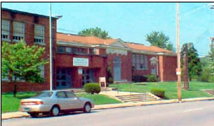
The school prior to rehabilitation.
