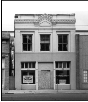
Commercial building prior to rehabilitation.
