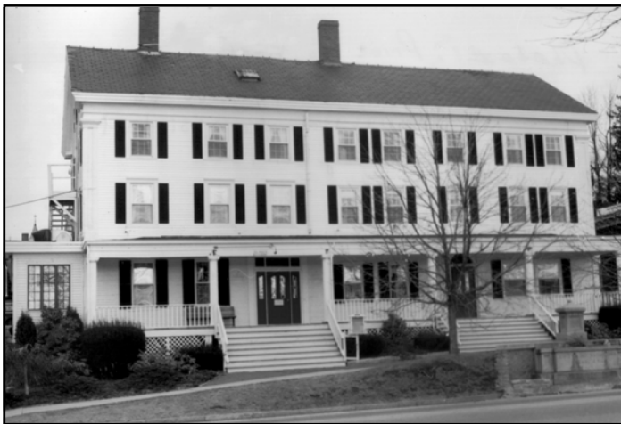
Tavern after rehabilitation before appropriate entrance installed.
