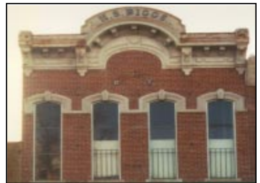
The second story of the primary facade showing non-historic fixed sash before rehabilitation.
