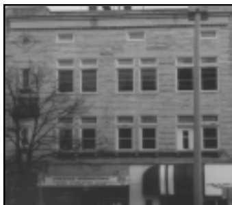
Before and after rehabilitation, one-over-one sash helped retain this commercial building's historic character.
