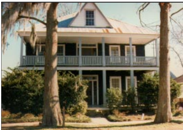
Before rehabilitation - simple historical balustrade.
