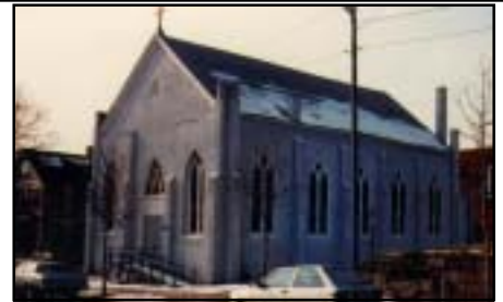
1858 Gothic Revival church building prior to rehabilitation.
