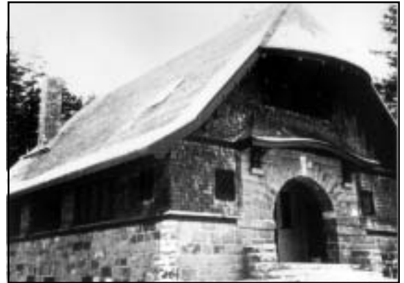
Shingle-Style church. North and east elevations after rehabilitation.
