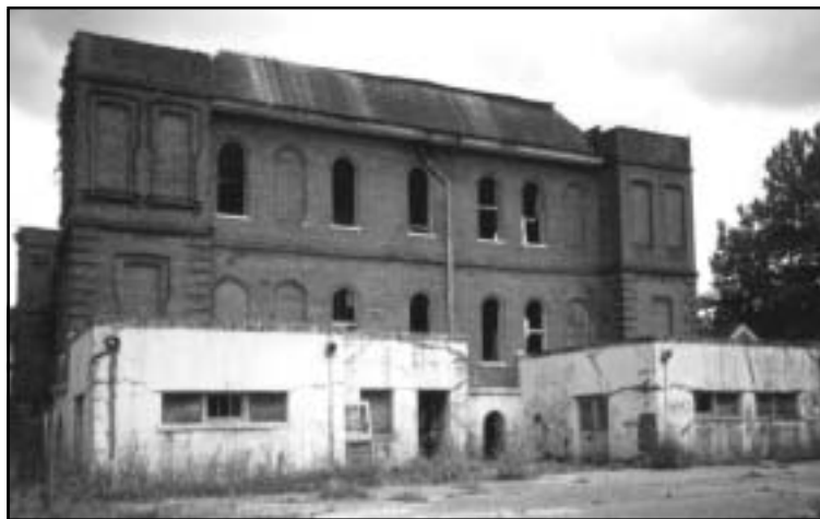
The rear elevation of the school building before the removal of the two later, non-significant additions.
