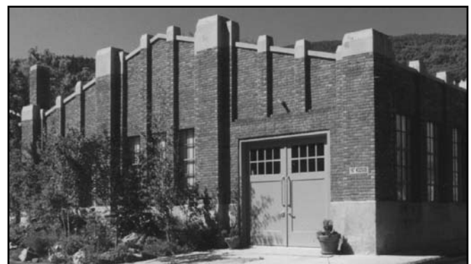
The owner chose to duplicate the original garage doors. The new doors preserved the industrial character of the historic building.
