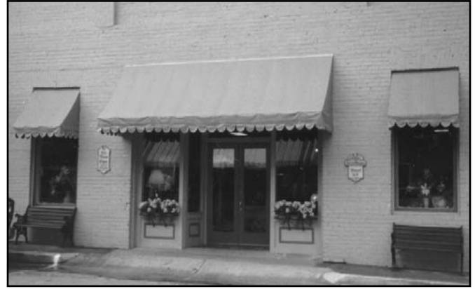
During rehabilitation the owner infilled the garage door opening with a storefront reminiscent of those used in the early-20 th century, which is not in keeping with the historic character of the building.
