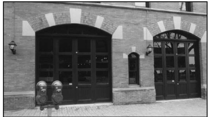
The design of the replacement doors is articulated with multi-paned units, maintaining the historic character of the building.
