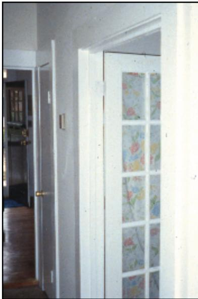
Interior Detail. The new wall added to create a private master bedroom is easily reversible. In addition, the glazed doors retain a sense of the light filled room when kept in an open position.
