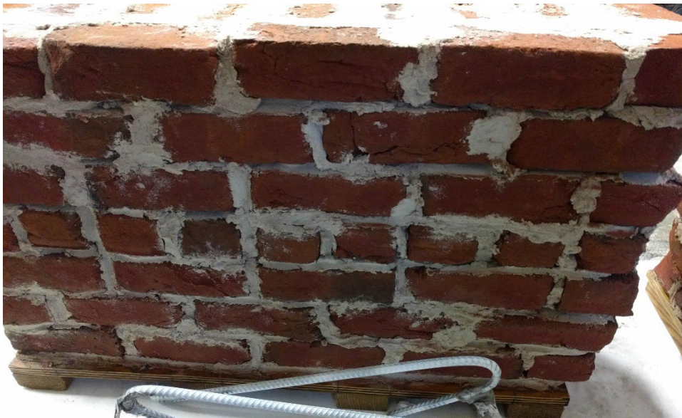
Figure 15. Photograph of Wall A exterior after treatment.
