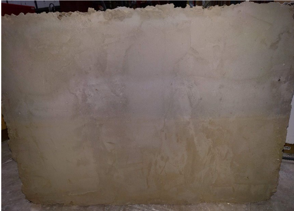
Figure 33. Photograph of Wall K exterior after treatment.
