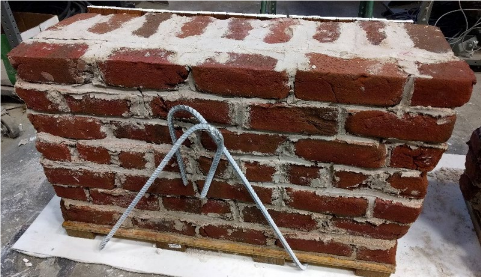
Figure 23. Photograph of Wall J exterior after treatment.
