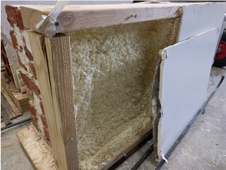
Figure 43. Photograph of Wall E cavity showing resilience of spray foam insulation.
