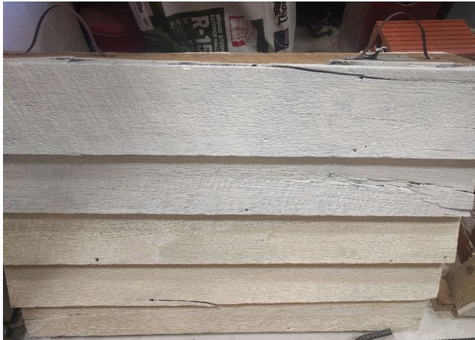
Figure 35. Photograph of Wall L exterior after treatment.
