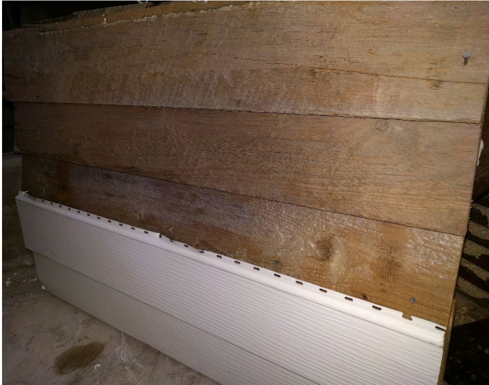
Figure 31. Photograph of Wall G exterior after treatment and disassembly.
