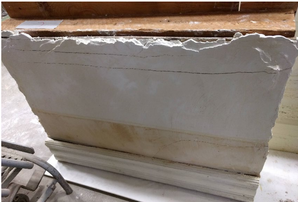
Figure 26. Photograph of Wall C interior after treatment.
