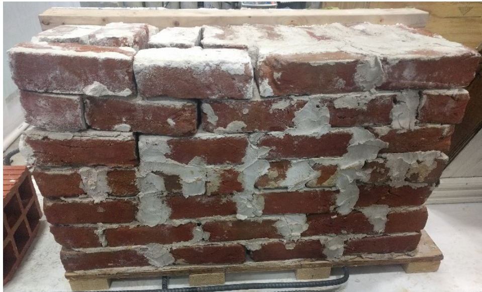
Figure 19. Photograph of Wall E exterior after treatment.
