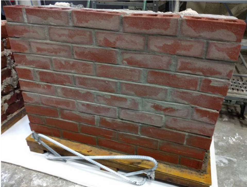
Figure 17. Photograph of Wall B exterior after treatment.
