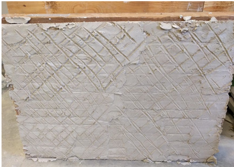
Figure 8. Plaster scratch coat with scoring allowed to dry.
