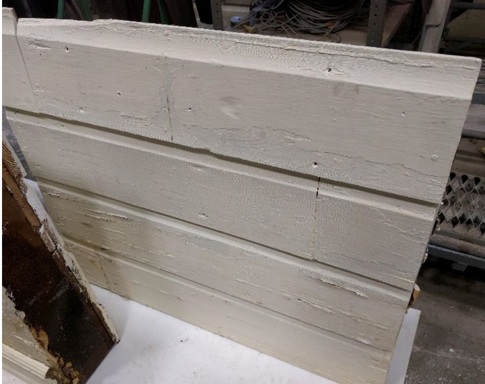
Figure 25. Photograph of Wall C exterior after treatment.
