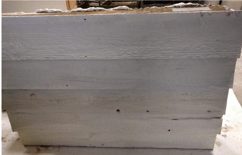
Figure 29. Photograph of Wall F exterior after treatment.
