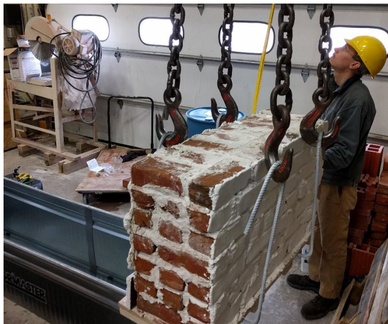
Figure 11. Lifting Wall A into position at the beginning of Test 1.
