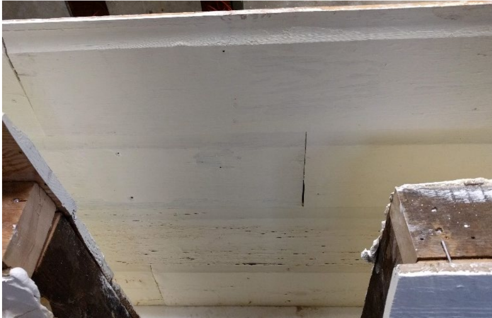
Figure 27. Photograph of Wall D exterior after treatment.
