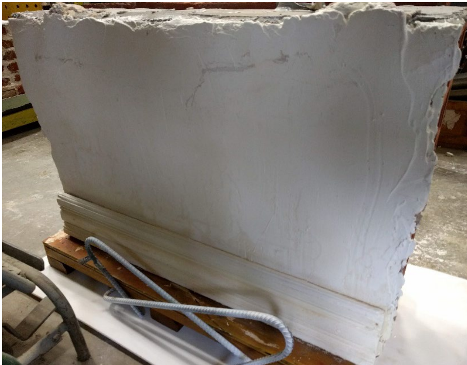
Figure 18. Photograph of Wall B interior after treatment.
