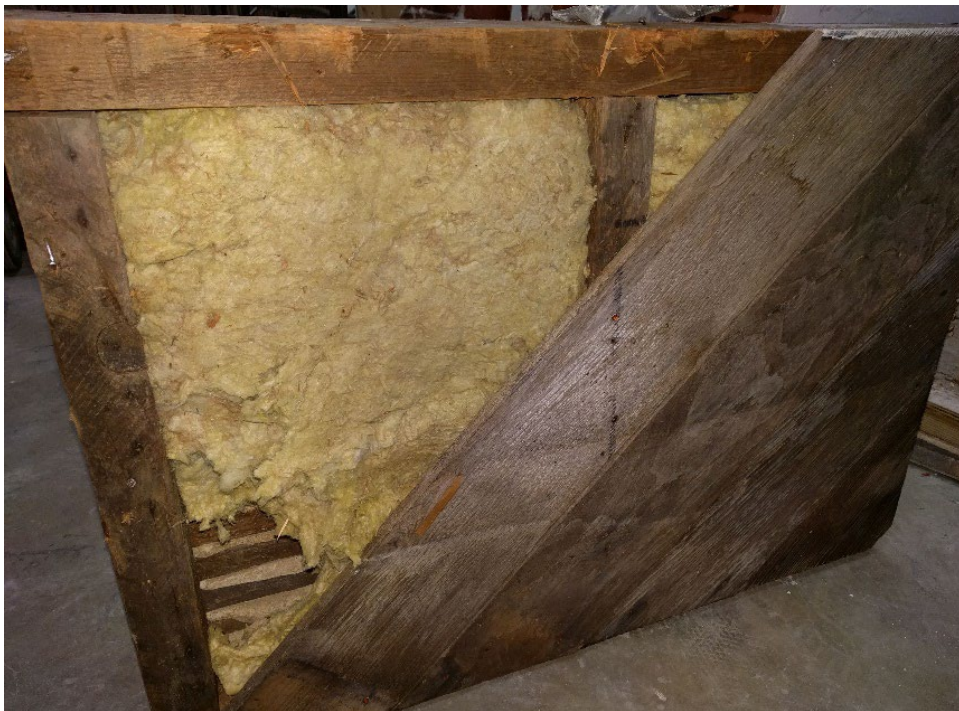
Figure 32. Photograph of Wall H cavity after treatment and disassembly.
