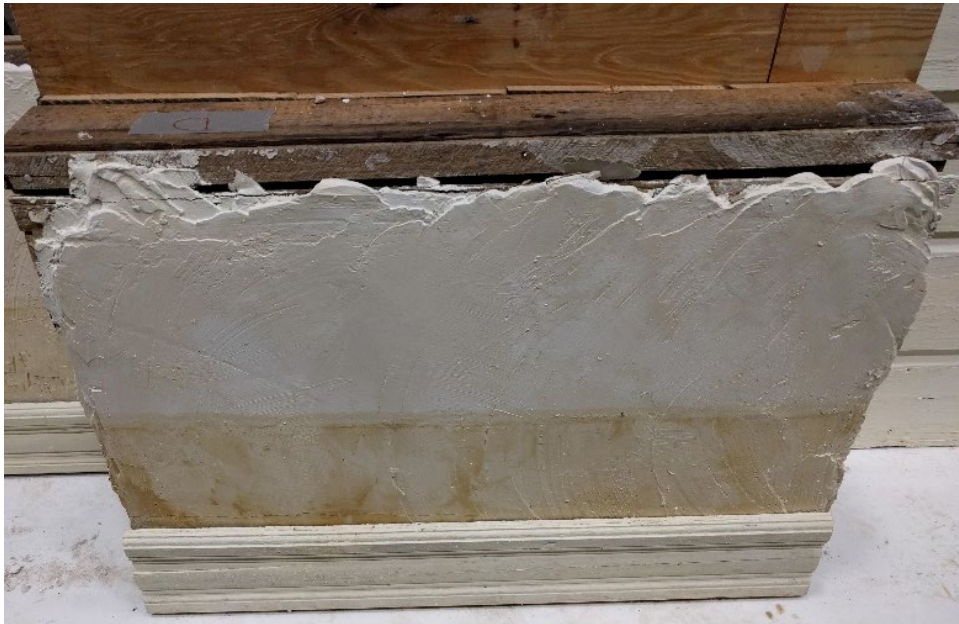
Figure 28. Photograph of Wall D interior after treatment.
