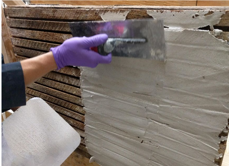
Figure 7. Plaster scratch coat application.
