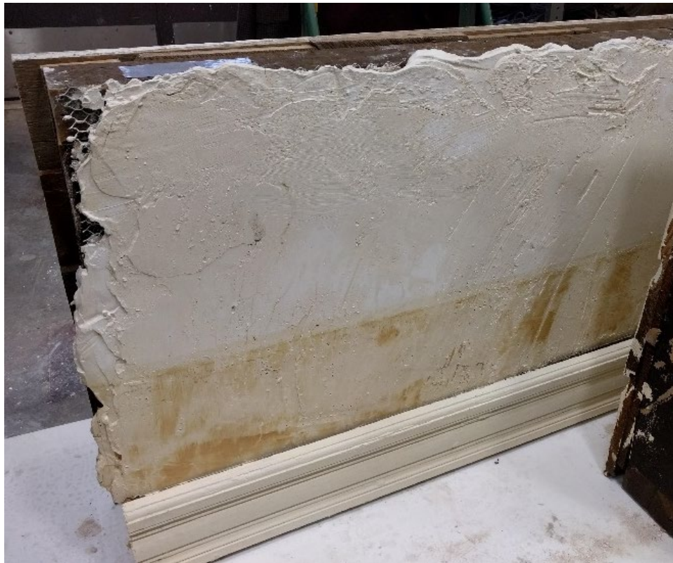
Figure 30. Photograph of Wall F interior after treatment.
