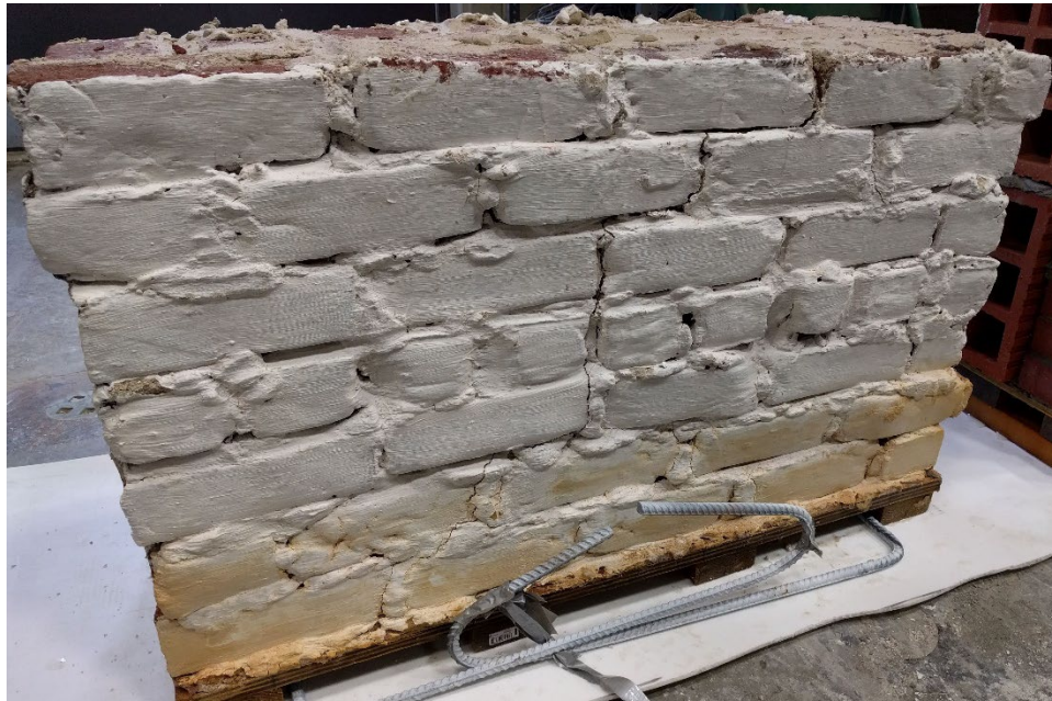
Figure 21. Photograph of Wall I exterior after treatment.
