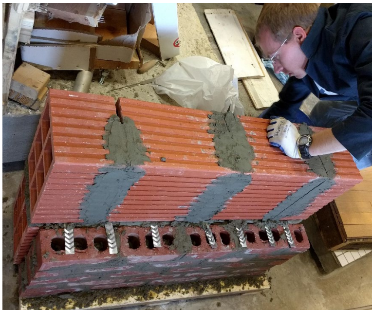
Figure 4. Construction of Wall B.
