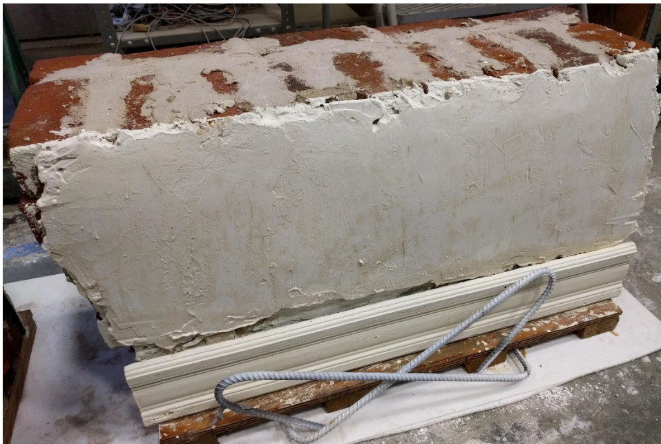
Figure 16. Photograph of Wall A interior after treatment.
