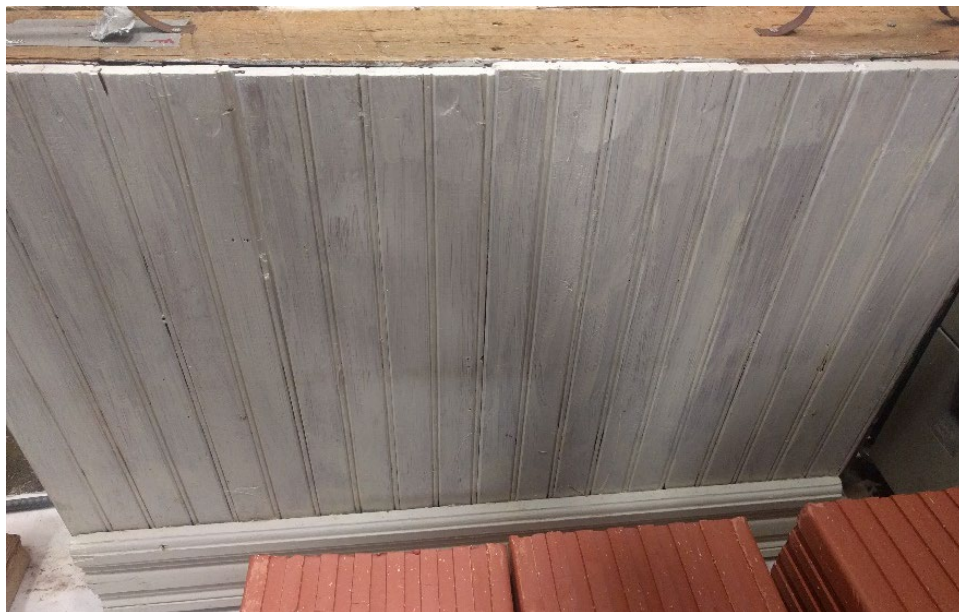
Figure 36. Photograph of Wall L interior after treatment.
