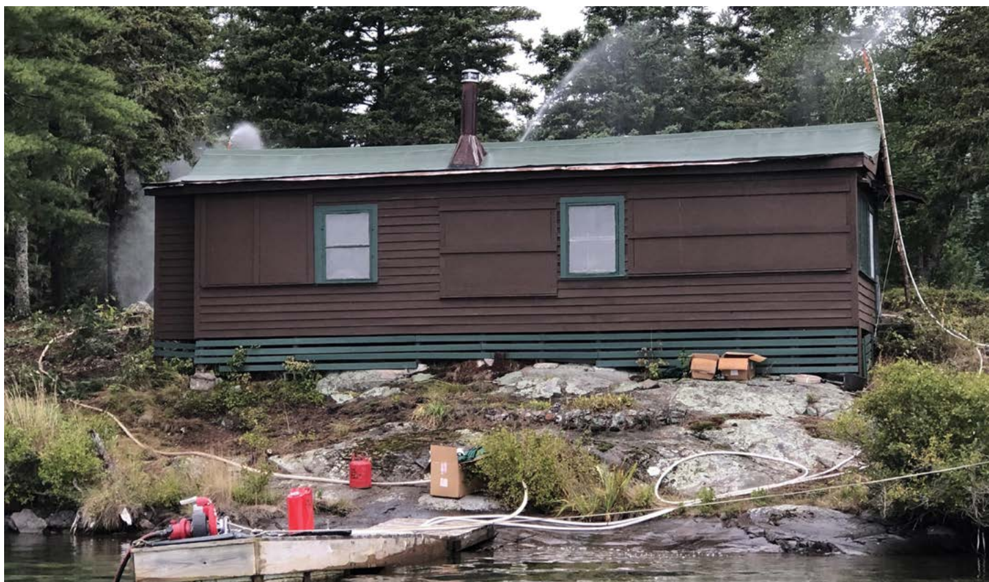
Figure 30: A temporary exterior sprinkler system that draws from an independent water source using a portable pump (visible at the end of the dock) has been installed ahead of an approaching wildfire to increase the humidity immediately around the building. Water-based sprinkler systems can help lower the probability of ember-caused ignition or autoignition. However, there are no national standards for such systems, and they rely on maintaining a continuous water supply and reliable power. Photo: Liz Valencia / NPS
