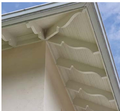
Figure 18: Existing vents should be covered with 1/8-inch or smaller corrosion-resistant noncombustible mesh, shown here in comparison to more open mesh designed to block vegetative debris or wildlife (left), or replaced with wildfire-rated vents. When open eaves are important character-defining features, treatment alternatives should be explored to retain their appearance while reducing their wildfire vulnerability (right). Photos: (left) Ethan Turpin / Santa Barbara County Fire Safe Council; (right) NPS
