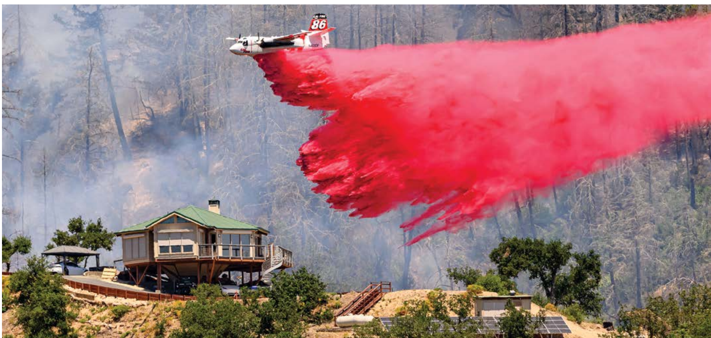
Figure 31: Aerial fire retardant drops can coat a building during a wildfire response. These chemicals can cause staining, efflorescence, and swelling of fragile, porous historic building materials. Post-fire removal is time-sensitive, but access to the site and the water supply needed may be unavailable in the days following a fire, increasing the risk of permanent damage to the building. Photo: Josh Edelson / Getty Images
