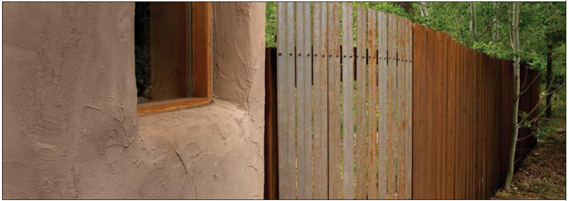
Figure 13: Noncombustible fencing within Zone Zero breaks continuous fuel paths such as those created by a traditional wood fence attached to a building or under roof overhangs. In this example, metal fencing evokes the appearance of the wood fencing beyond. Photo: Boulder County Wildfire Partners
