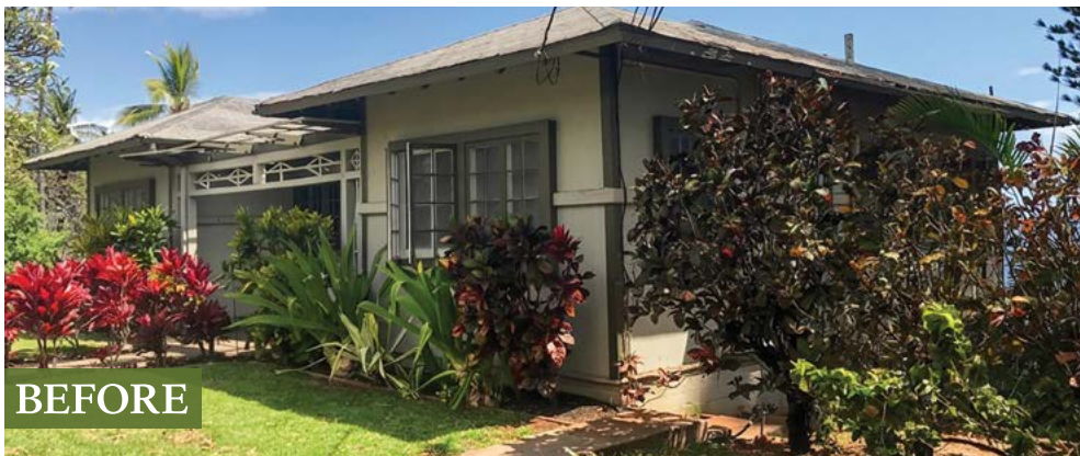
Figure 28: This vernacular wood building survived the devastating August 2023 Lahaina wildfires. Prior to the fire, mulched foundation garden beds were replaced with river rock below the roof overhang, and trees and other vegetation were removed. On a very small lot, a wider defensible space was effectively created on three sides of the building by virtue of the paved road in front, an empty lot on one side, and the ocean 15 feet away behind it.
