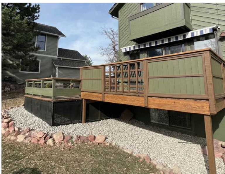
Figure 21: Decks and other projecting building features can be partially mitigated with gravel or rock mulch below and surrounding them, plus, depending on the deck height, ember-blocking mesh. Windows near the ground may require additional fortification, such as safety glass and metal screens with ember-blocking mesh. Photo: Fire Ready Exteriors
