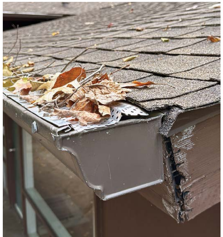
Figure 26: Routine inspections and maintenance to remove vegetative debris and close gaps in the building exterior are important for wildfire resilience and may help prevent the need for extensive building repairs later. Photo: NPS
