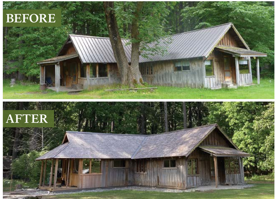
Figure 28: This vernacular wood building survived the devastating August 2023 Lahaina wildfires. Prior to the fire, mulched foundation garden beds were replaced with river rock below the roof overhang, and trees and other vegetation were removed. On a very small lot, a wider defensible space was effectively created on three sides of the building by virtue of the paved road in front, an empty lot on one side, and the ocean 15 feet away behind it.
