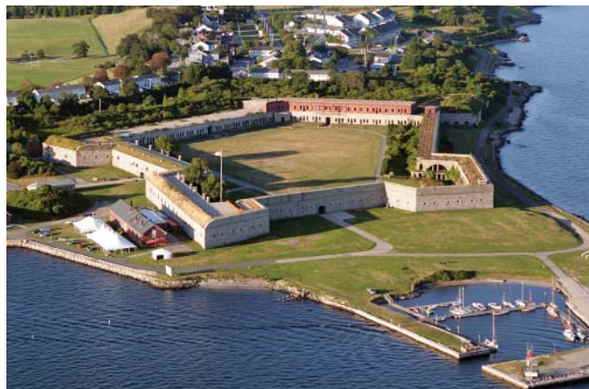
Begun circa 1824, the pentagonal-plan Fort Adams is situated in Newport, Rhode Island, on the Narragansett Bay. Built of shale and Maine granite and regarded as a milestone in coastal fort construction at the time, Fort Adams was conveyed to the state and offers interpretive programs for the public. Credit: Billy Black, Newport, Rhode Island
