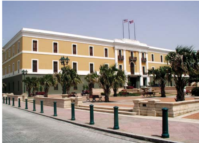
Built between 1854 and 1864 as barracks for the Spanish infantry, the Cuartel de Ballaja in Old San Juan, Puerto Rico, was conveyed to the commonwealth for public use. It houses a museum and state offices. Credit: Frank Miele, National Park Service, Southeast Region
