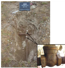
RIGHT: Crane valve on the pipe distribution system. Manufacture of this particular valve began in 1902.
