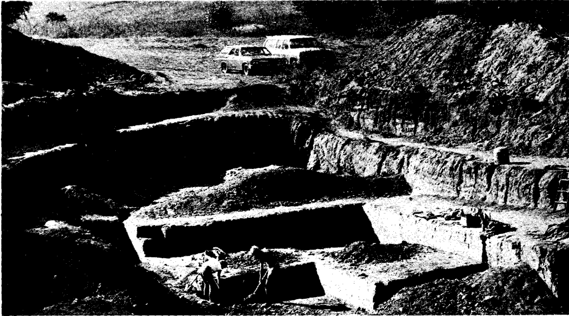
Figure 18. Held Creek Watershed, Iowa (Plymouth County). The uppermost two steps were opened with a backhoe. Below, the excavation is being completed at about a 16 ft. depth. Courtesy Luther College, Decorah, Iowa.
