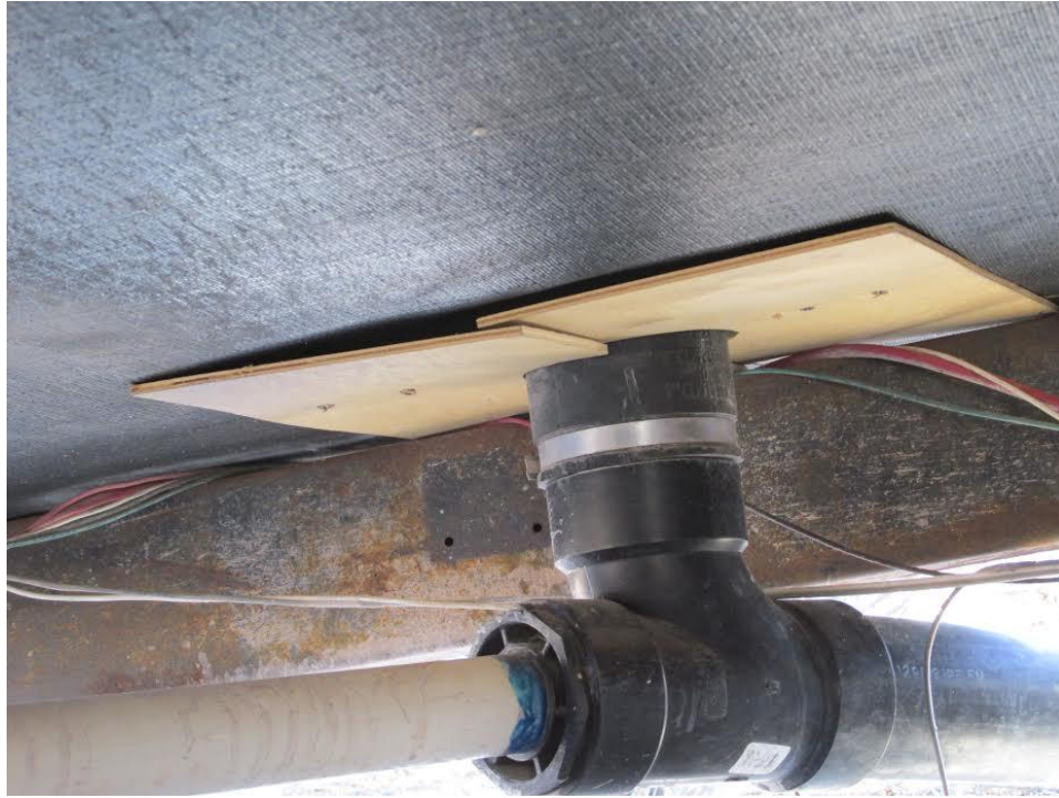
Figure 28: The underside of trailers should be rodent proofed prior to human occupation. Figure credit: NPS Figure.
