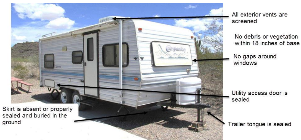
Figure 13: External points to evaluate on a mobile trailer: check that all exterior vents are screened, ensure no gaps exist around windows, no debris or vegetation exists within 18 inches of the base of the trailer, utility access door and trailer tongue are sealed, and the trailer skirt is absent or properly sealed and buried in the ground. Figure credit: NPS Figure.
