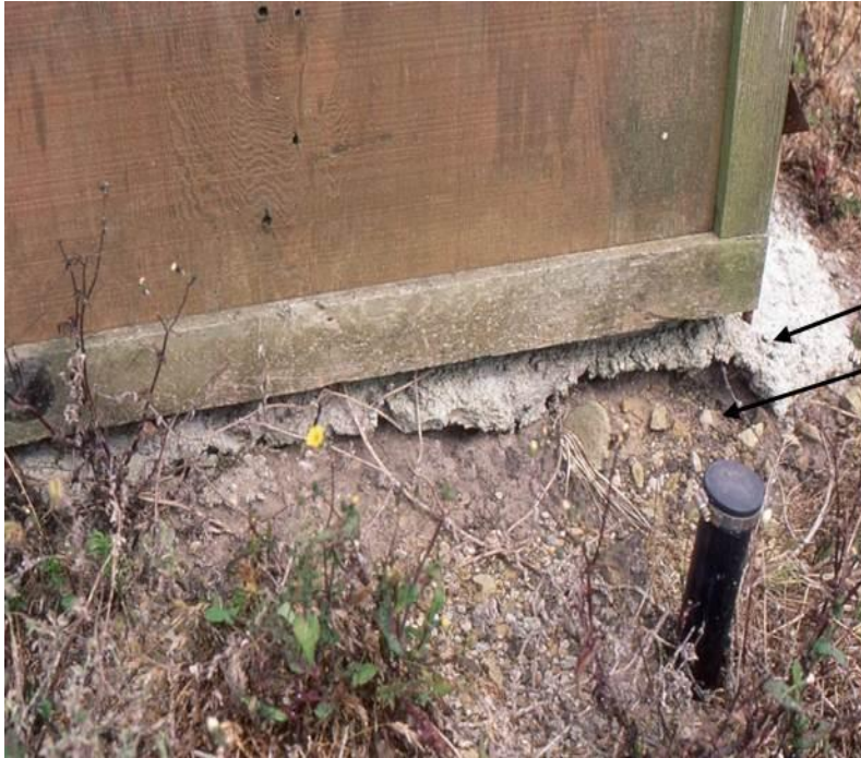
Figure 6: This foundation has a gap between the foundation and building providing potential rodent access into the building. Figure credit: NPS Figure.
