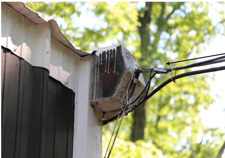
Figure 12: Electrical cables covered with \frac{1}{4} " hardware cloth at the cable/roof junction to exclude rodents at the cable entry point. Figure credit: NPS Figure.
