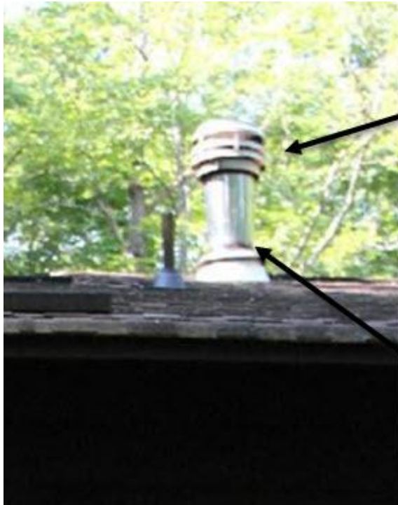
Figure 11: This properly installed chimney and vent pipe has a rodent proof cover. Evaluate the chimney and vent pipes on the roof to ensure that they are covered and flashing is tightly sealed to the roof. Also evaluate the roof for holes, gaps, or low points where water might pool and provide a water source to rodents. Figure credit: NPS Figure.
