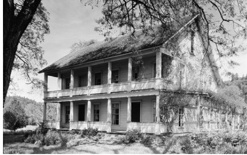
Applegate Pioneer House in 1934. Courtesy of the Library of Congress.
