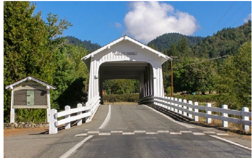
Grave Creek Bridge (stop C-12).
