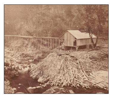
Figure 61. As companies built Oregon's first railroads, they built accompanying infrastructure to support the construction of those railroads. Here, the Oregon Steam Navigation Company's Eagle Creek Sawmill, near the Columbia River's Cascades rapid. Photograph by Carleton E. Watkins, 1867.
