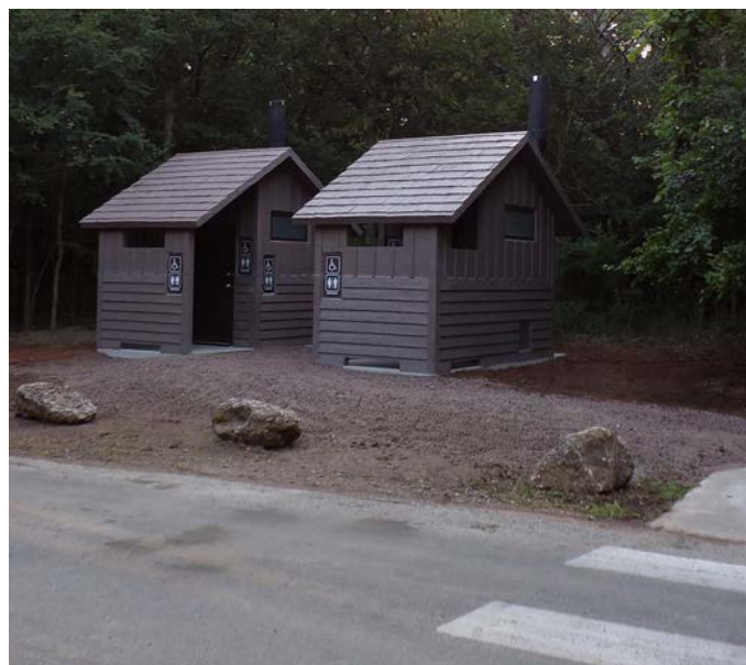
New vault toilets at Panther Falls / NPS Photo
