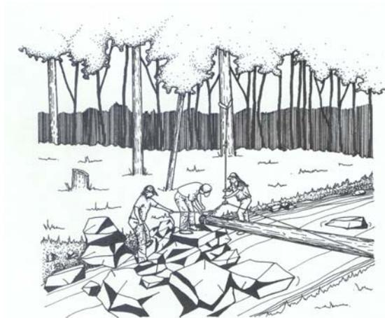
Rigging systems are most appropriate when there is a considerable amount of work to do at one site—such as when constructing a bridge, retaining wall, steps, or shelter. On this type of project a crew will not want
