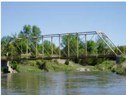
The Borman Bridge is located 2.3 miles south of Valentine, past the town cemetery. Borman Bridge marks the western boundary of the national scenic river. Built after an ice jam swept away 14 bridges in February 1916, Borman is a 131 feet long pin-connected Pratt through truss. A plaque fastened on top of the bridge's end reads, "1916, The Canton Bridge Co. Builders, Canton, Ohio". Borman along with Allen (Bell),
