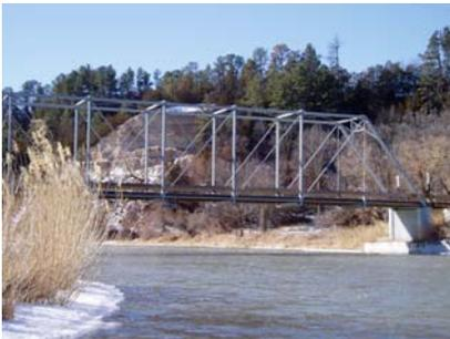
Located 4 ½ miles south of Sparks, Nebraska, this bridge was restored in 2003. An 8-panel, pinned Pratt through truss, Allen was built in 1903 by the Canton Bridge Company. The river ford was once called Bell Crossing. At 188 feet it is the longest single-span bridge on
