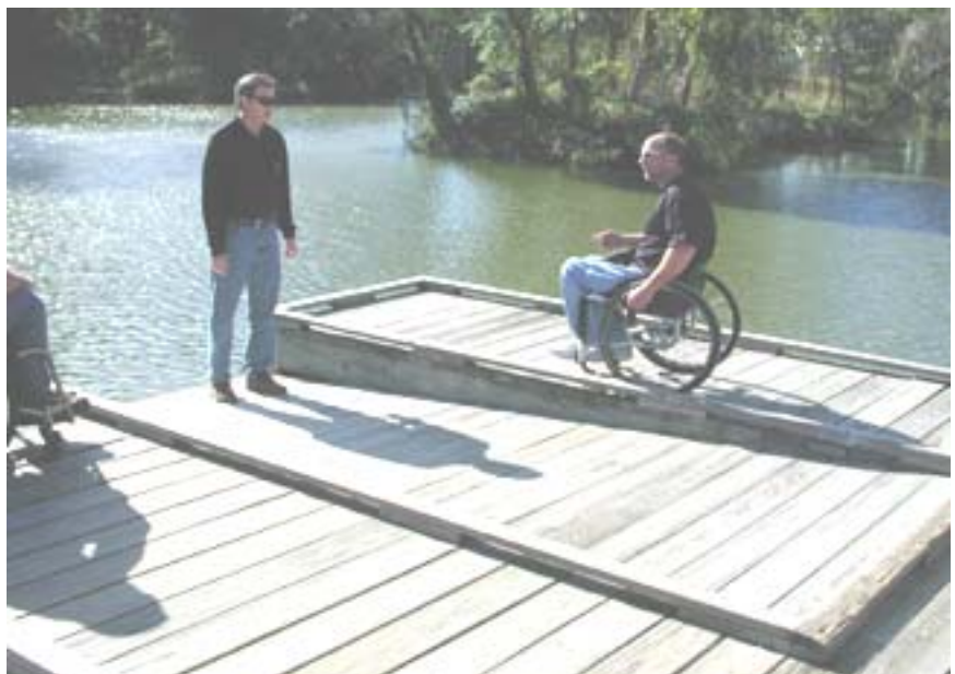
Photos 3C, 3D: ADA accessible wooden floating launch has two tapered ramps that allow canoes to slide up onto the deck
