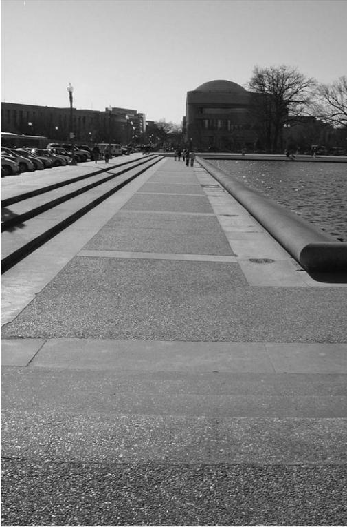
Paving composed of limestone and concrete, contrasting in color and texture, articulates the wide sunken walk surrounding the reflecting pool. View looking west. (CLP file "plaza and walk along S side pool" Feb. 24 2006)
