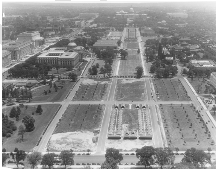
Figure 4. American elms newly planted between 12 th and 14 th Streets on the National Mall, summer 1935. Possible Civilian Conservation Corps encampment in the center. (from MRCE; CLP file "Gov buildings and Mall 1935")
