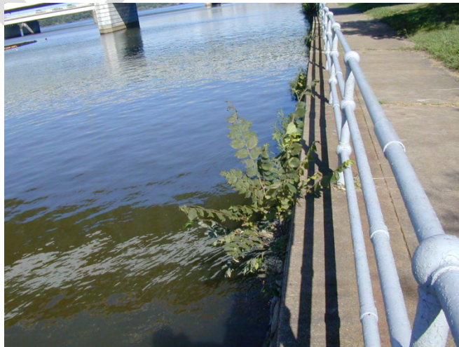
Figure 53. Seedling American elm growing out of the seawall in East Potomac Park..
