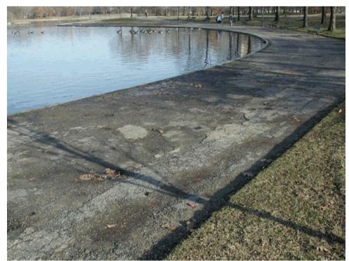
The walk circling the lake has lost much of its gravel, and the exposed asphalt is deteriorated. (Jan. 2007; CLP file)
