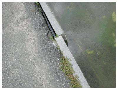
The granite walls that line the lake and create a curb along the lakeside walk occasionally pop from their anchors. This image also shows the heavy growth of algae that had developed on the water's surface by mid-June 2007. (CLP file)
