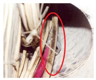
Figure 6. Dark rub marks (circled in red) on white electrical wire from mice using the wire to travel around the museum. (Thomas Parker, PhD, MuseumPests.Net)
