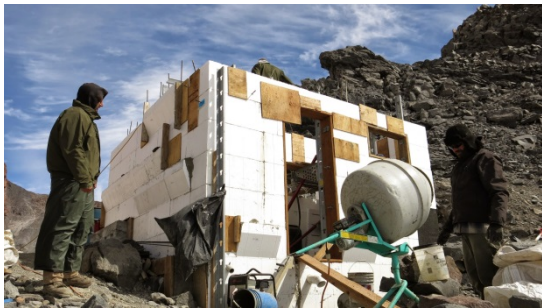
Figure 11 New toilet construction at Camp Muir
