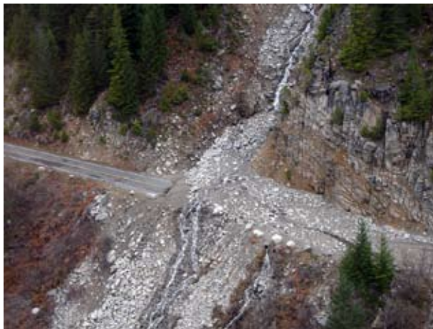
A landslide on Steven's Canyon Road.
