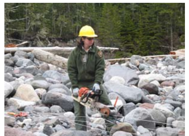
Trail crew at work after the flood.
