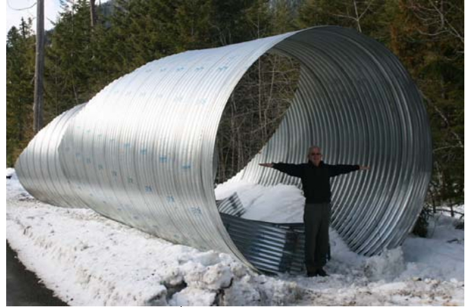
The 12-foot culverts ready for installation
