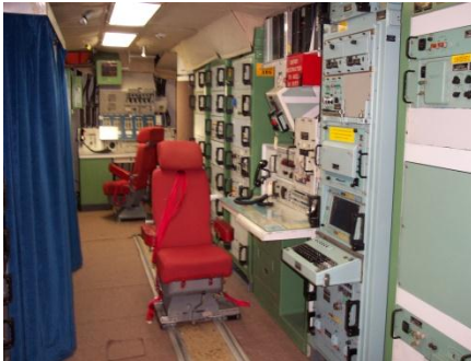
Launch Control Center Delta-01
