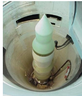
Launch Facility Delta-09
