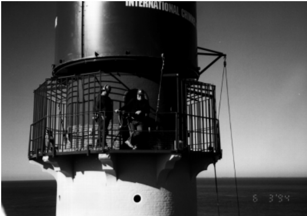
Figure 6. During the restoration, this ‘Campbell Soup Can’ was installed over the lantern room in order to protect restoration efforts from the environment.
