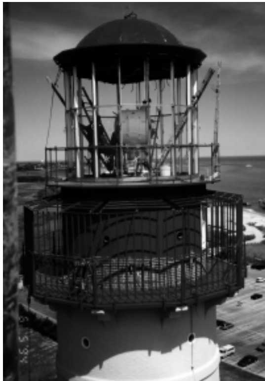
Figure 9. The refurbished roof is replaced on the lantern room. The fit is almost exact.
