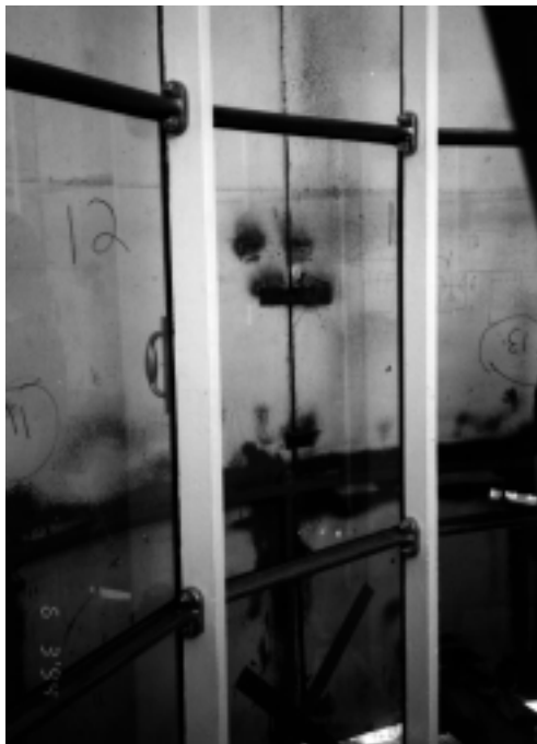
Figure 7. Inside the lantern room, the mullions have been reworked and reattached to the stiles. New stainless steel bolts have been used to prevent corrosion and teflon tape has been used as a gasket between the bronze and the cast iron. Teflon washers also separate the bronze from the stainless steel bolt.
