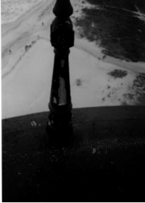
Figure 14. The handrail assembly has been removed and the ornate cast-iron post is ready for removal.
