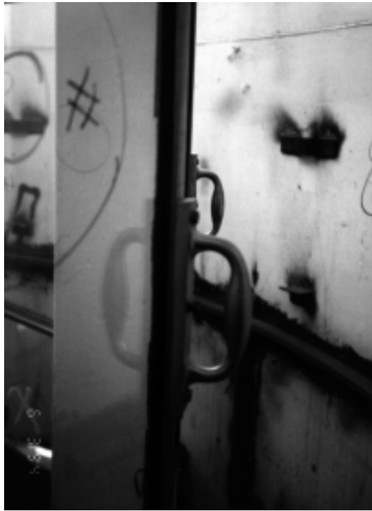
Figure 8. New hand holds were replicated to replace missing pieces. These exactly match the originals.
