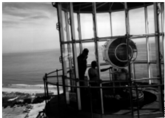
Figure 10. All glass is now in place and final preparations are made for the reopening.
