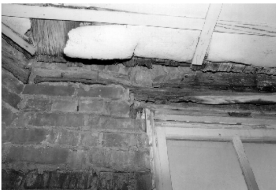
Figure 4 (left). Extensive interior finish deterioration in a lighthouse that had holes in the roof which were not repaired.
