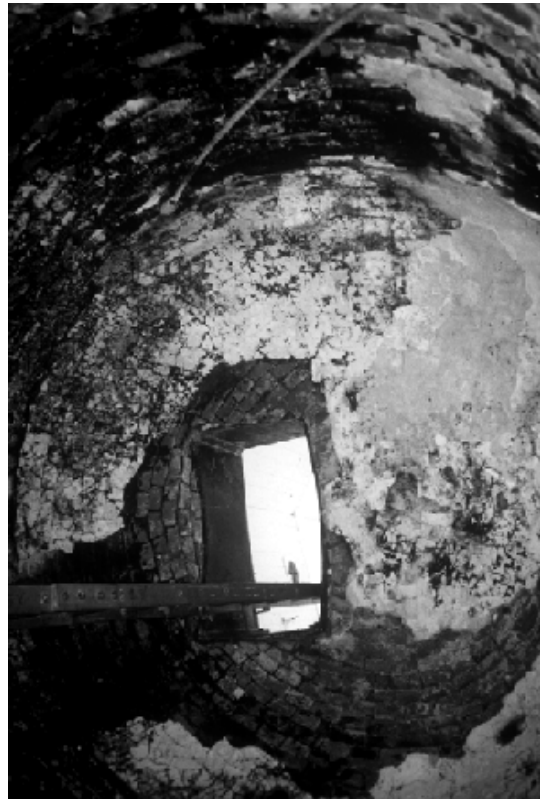
Figure 4 (left). Extensive interior finish deterioration in a lighthouse that had holes in the roof which were not repaired.
