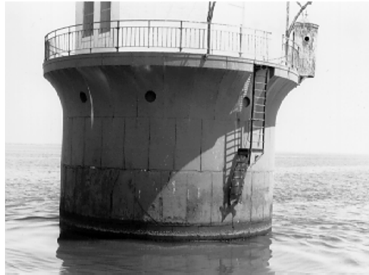
Figure 17. The cyclic pressure of the different rates of expansion and contraction of the exterior cast-iron plates and the interior brick lining of the caisson-style lighthouse has caused the cast-iron plates to fatigue and crack.
