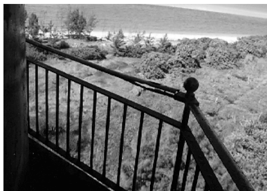
Figure 19. This handrail has been damaged by rust-jacking; rusting began between the two pieces of flat bar stock that formed the rail.
