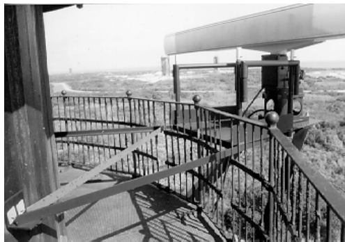
Figure 9. A modern range finder attached to the gallery deck using modern steel members.
