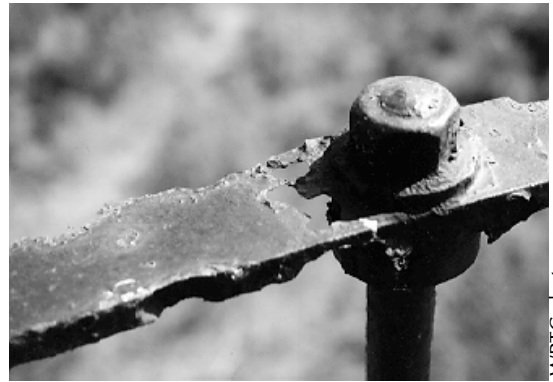
Figure 15. As corrosion attacked this steel handrail, wind and airborne sand eroded the loose and flaking surface rust.
