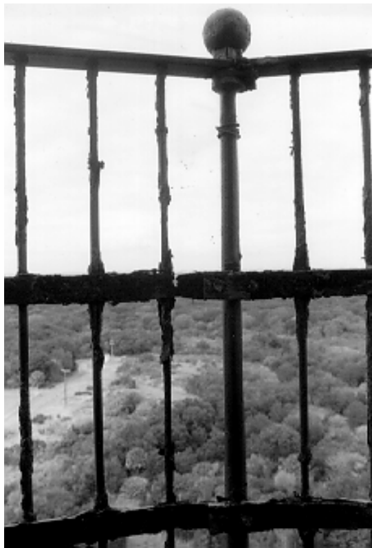
Figure 13. View of a steel railing where corrosion has occurred in distinct locations either because of variations in composition or localized failure of the coating system.
